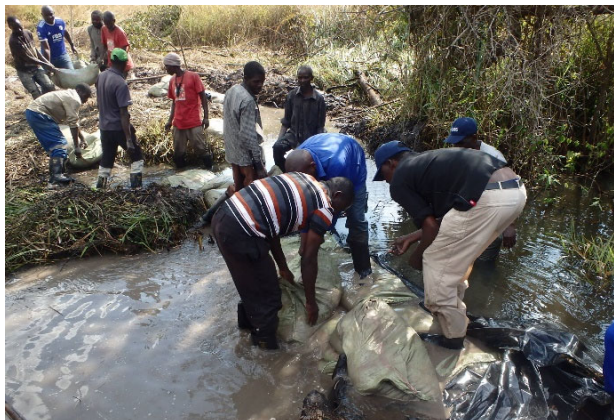
Farmers putting sandbags to make a temporary cofferdam (Mufulira District).
