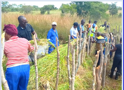
Practice of a simple weir construction (Central Province)
