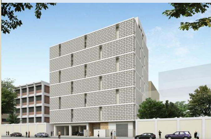
Conceptual Drawing. Project for Construction of Outpatient Facility at CUSPH (Grant Aid).
