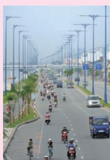
Saigon East-West Highway Construction Project (Courtesy of Koji SATO)
