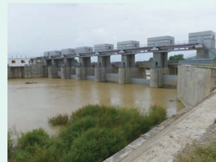
Headworks constructed upstream of the Phan Ri-Phan Thiet irrigation channel
