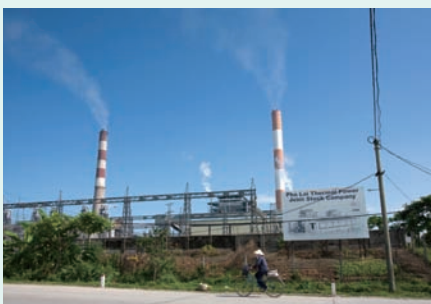
Pha Lai Thermal Power Plant Project
