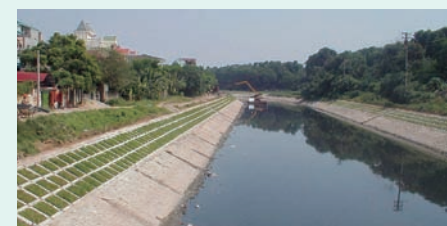
View of Completed Section of the To Lich River Improvement Works
