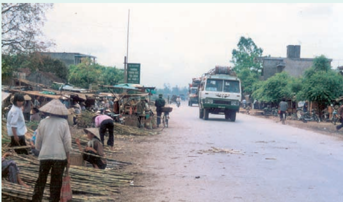
National Highway No.5 before improvement
