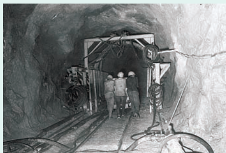
Excavation of the pressure tunnel
