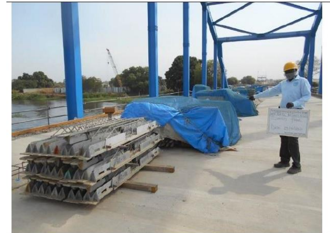
The scaffolding materials were properly arranged on top of the slab
