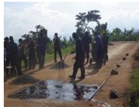
Part of road works are done by manpower
