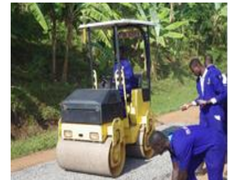
Partially using equipment like 1t vibration roller
