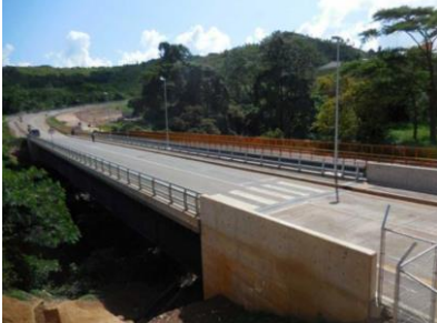
Bridge at Rusumo
