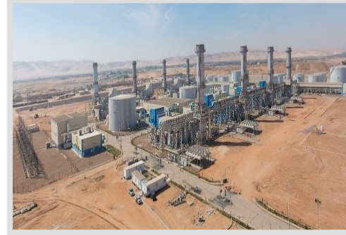
Assuit P.P adding 500 MW (Total capacity : 1500 MW)
