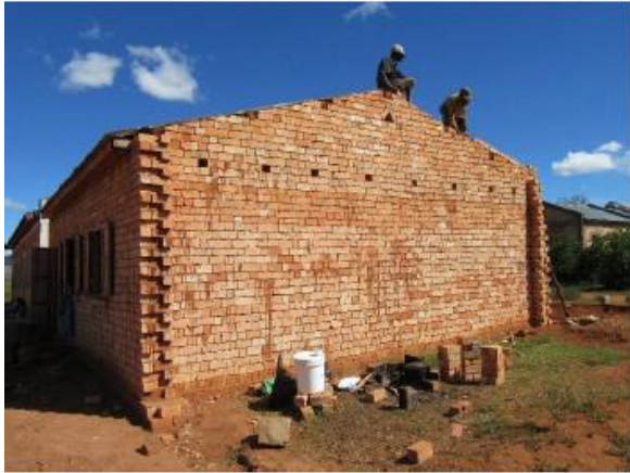
Construction of classrooms in Madagascar
