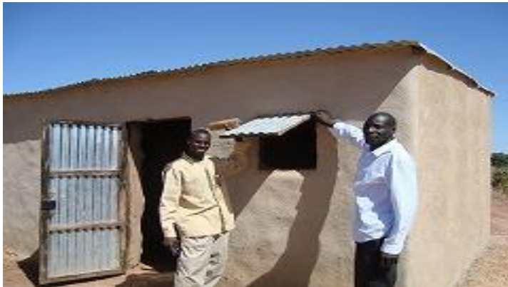
Housing construction for teachers in Mali
