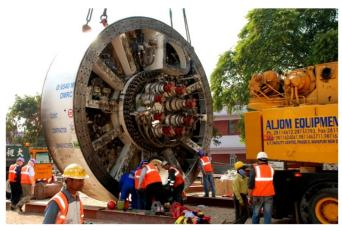
Assembling of a tunnel boring machine in Delhi Mass Rapid Transport System Project
