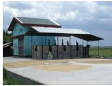
Warehouse & Solar Dryers
