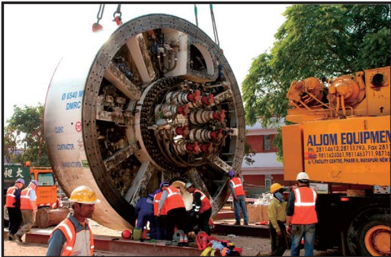
Assembling of a tunnel boring machine
