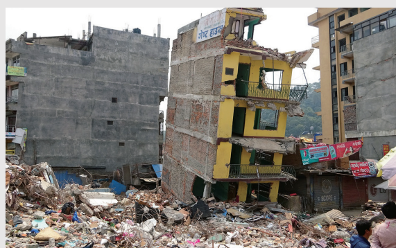
Damage of the 2015 Nepal Earthquake Disaster
