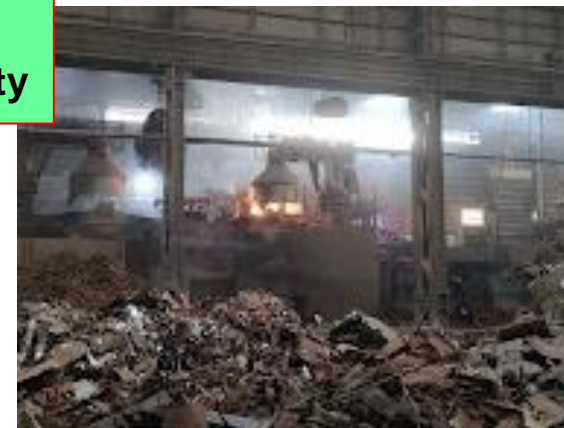
Steel Mills with gas purification systems
