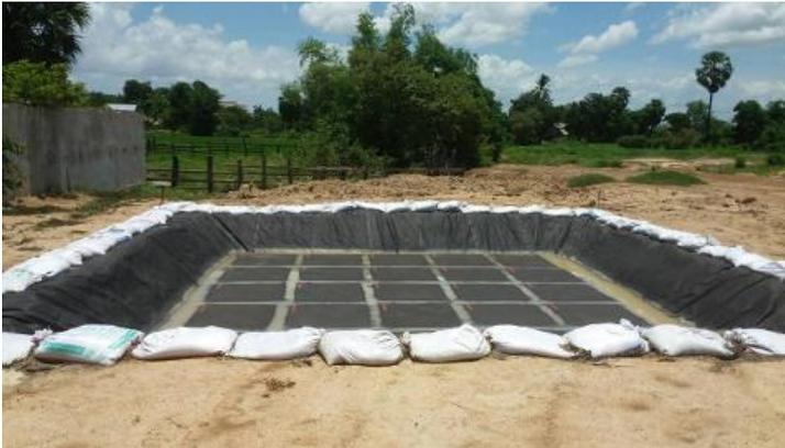
This lid will work effective for water losses by Evaporation.
