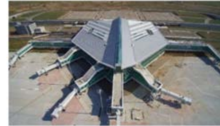
New Ulaanbaatar International Airport Operation Project
