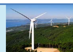
Wind power station
