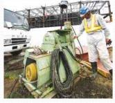
Shaft construction for manhole by special purpose machine by using concrete or steel casings.
