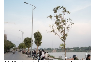
LED street lighting system with wireless network control, Minebea Mitsumi, Cambodia
