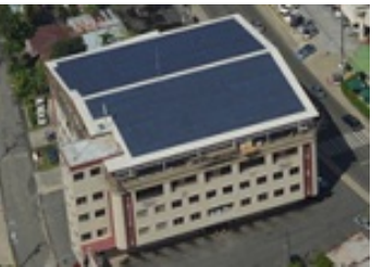
Installing solar PV system, PCKK, Palau and Maldives
