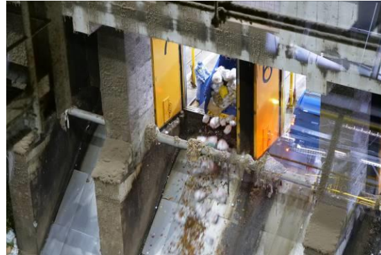
Photo 4-35 (1) Platform (Waste Pit)
