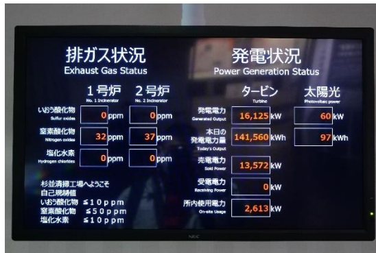
Photo 4-52 Disclosure of Exhaust Gas Status at Suginami Incineration Plant
