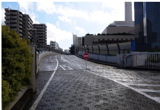
Photo 4-32 Facility Entrance for Waste Collection Vehicles
