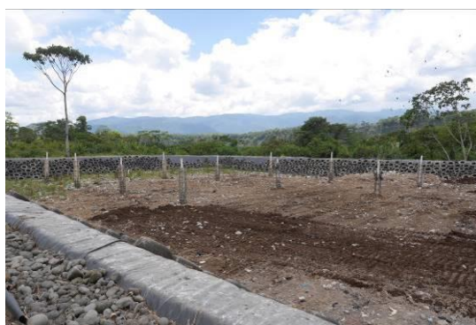
Photo 4-72 Appearance of the Landfill
