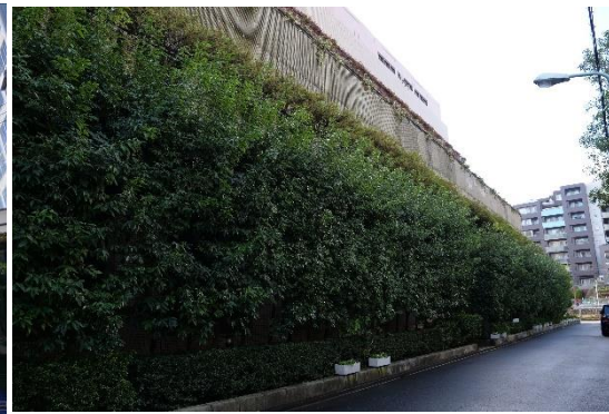
Photo 4-31 Green Exterior Walls
