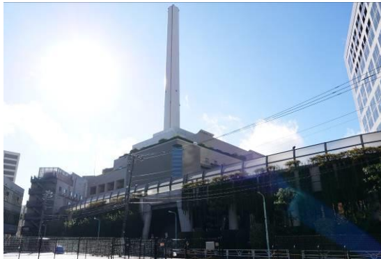
Photo 4-30 Outer View of Incineration Plant
