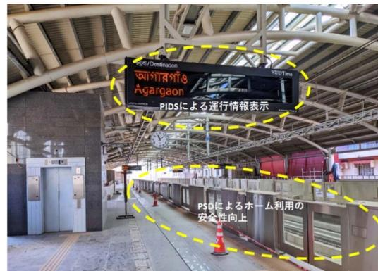
(ii) Example of ensuring accessibility for station and rail users: Passenger Information Display System (PIDS), and Platform Screen Door (PSD)
