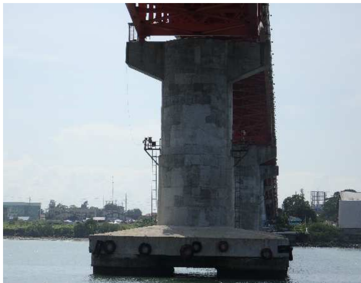
Photo11. Condition of the bridge piers
