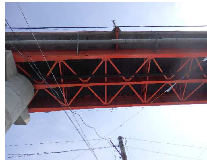
Photo12. Condition of the bridge girder
