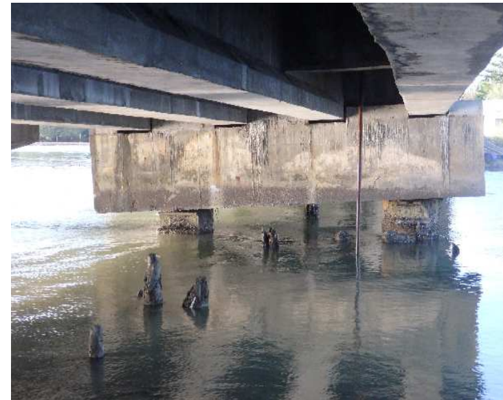
Photo10. Slope in the substructure
