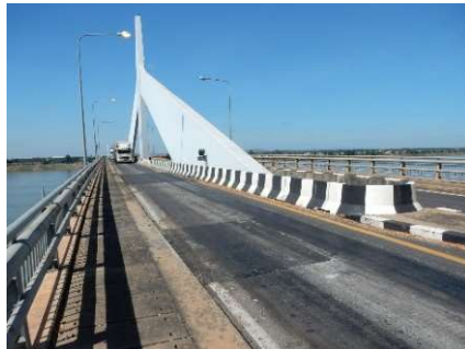
舗装表層打換
