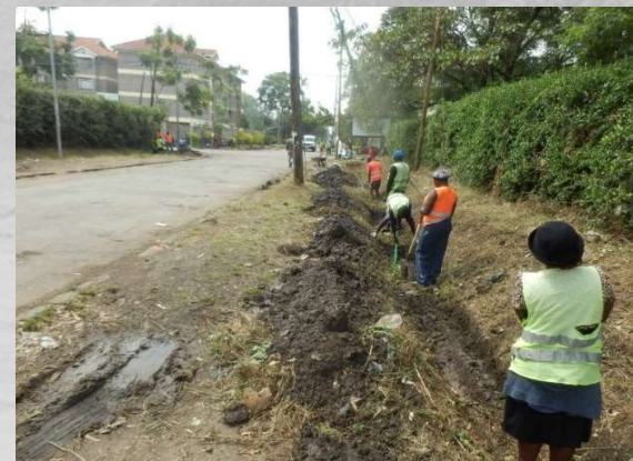
Ditch cleaning by PBC contractor
