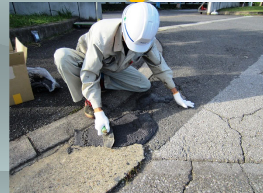
Use a metal trowel to rub against the road steps
