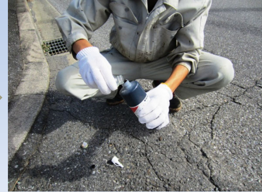
Put the hardener into the main bottle
