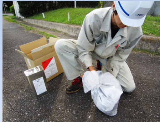
Mix while holding the aggregate bag
