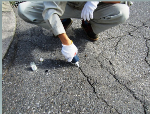
Inject into cracks within 10 minutes
