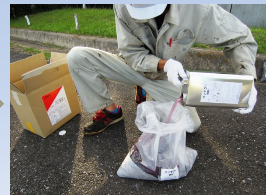
The resin is put into the aggregate bag after mixing.
