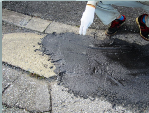
Apply anti-skid aggregate before hardening
