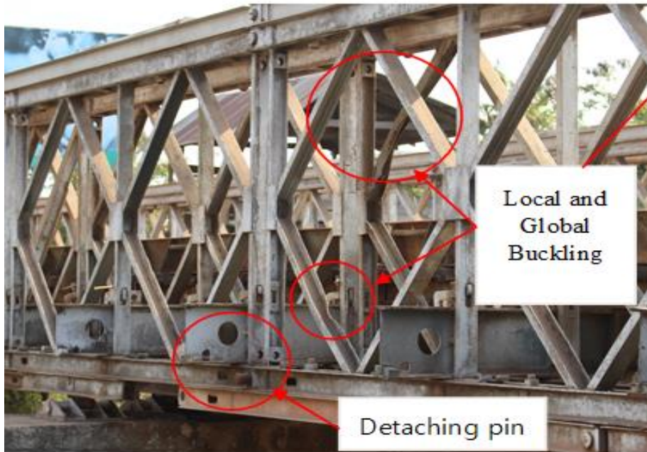
Loosened by corrosion and detaching pin
