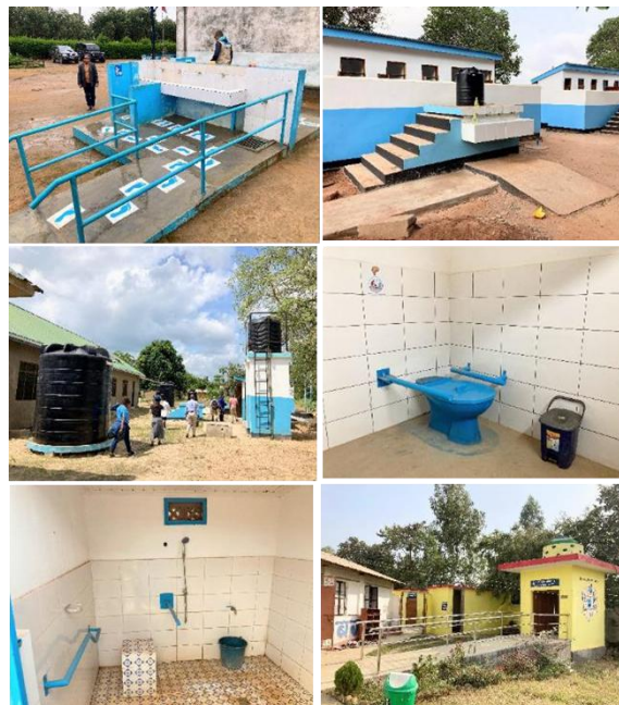
Figure 8: Examples of improved WASH facilities in schools
