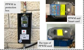
**The PPWM procured is ultrasonic type smart meter with a function of LoRa technology.** Twelve vending stations (VS) (Figure 13) were set up at convenient locations where customers could buy credits to recharge the meter. Through the Gateway and LoRa technology all PPWM could communicate remotely with PPWM server and PPWM customer database.
