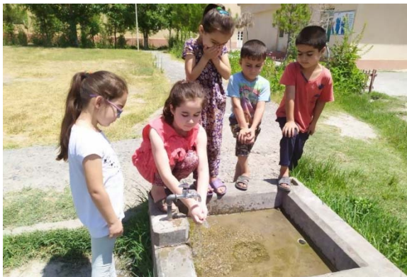
Picture 11: Water supply conditions after installation of water meters
