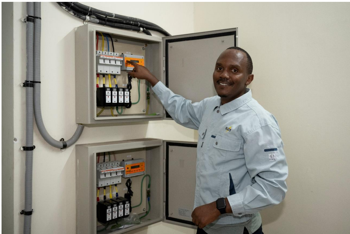
Photograph 2: Mugarura with the Otowa lightning protection devices.
