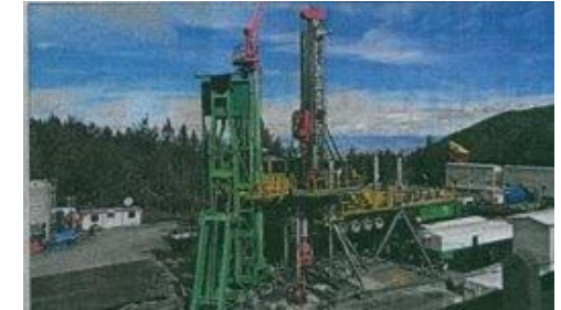
Geothermal Power survey at Chachimbiro plant
