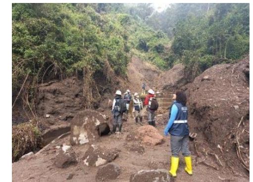
Survey of Landslide at La Gasca, Quito
