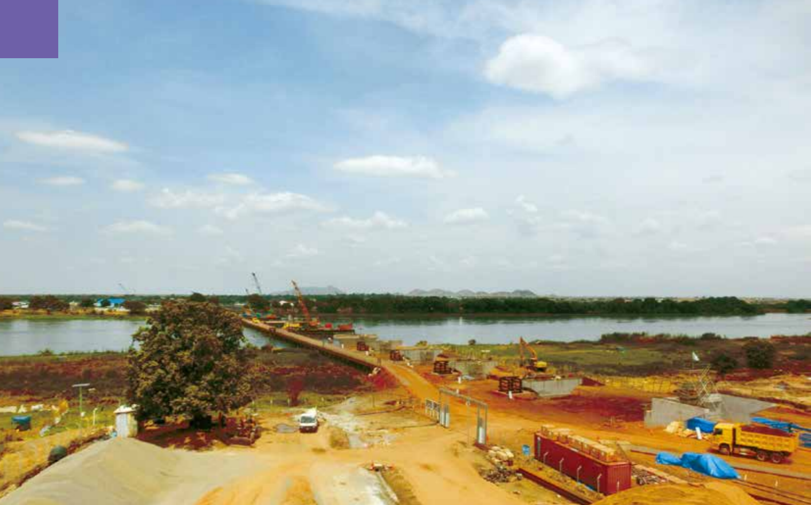
Photo: Dai Nippon Construction
