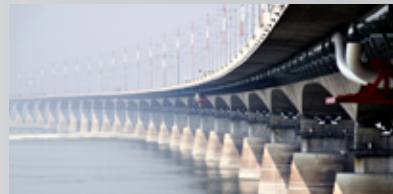
Jamuna Bridge in Bangladesh
