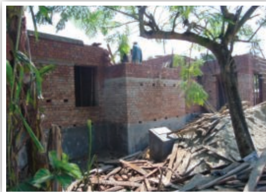
Construction is under way of Old Women resident building
