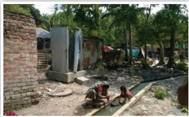
Before constructing Drainage system
