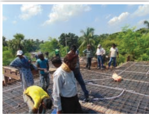
Construction is under way of Old Women resident building
