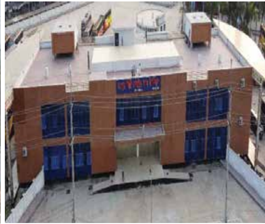
Constructed Bus Terminal at RpCC
