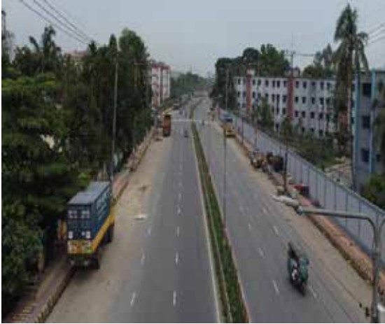
Constructed Port Connecting Road at ChCC
