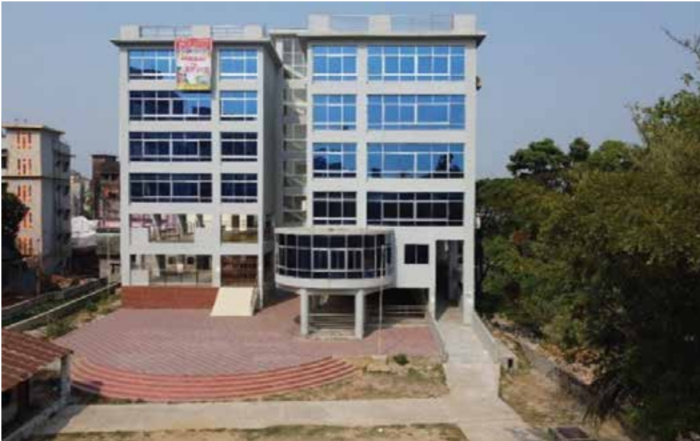
Constructed School Building Cum Cyclone Shelter
