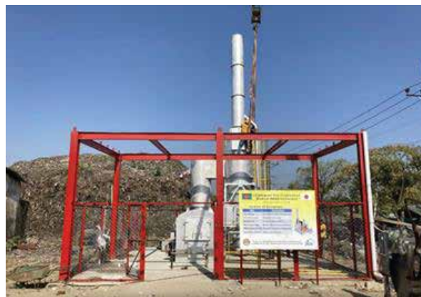
Installation of small incinerator (4, January 2022)
