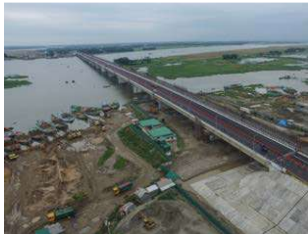
Gumti Bridge (Photo: JICA)
