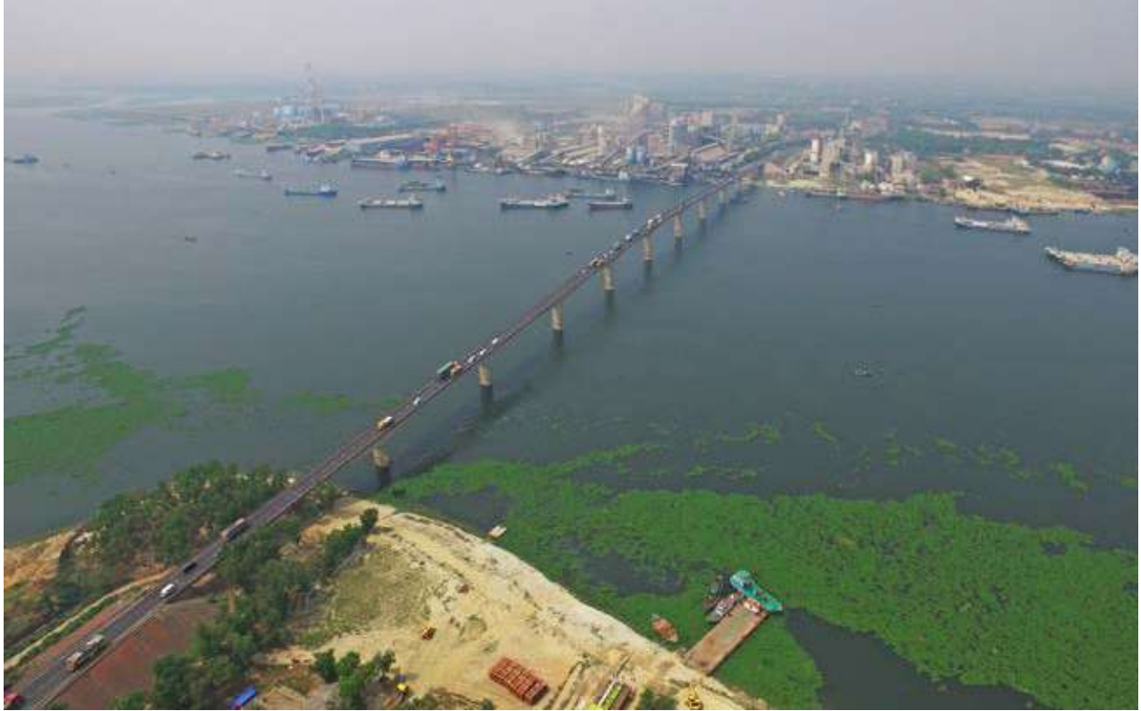
Meghna Bridge (Photo: OSJI Joint Venture)
