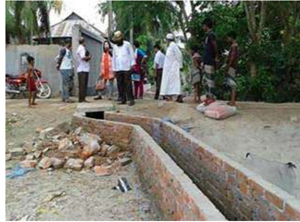
Irrigation canals constructed by the village committee project (Photo: JICA)
