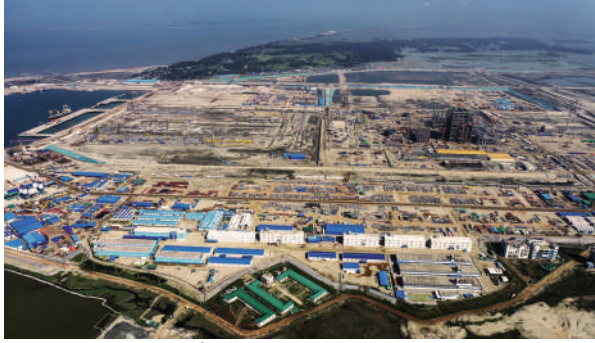
Construction status of Matarbari Ultra Super Critical Coal-Fired Power Plant (Photo: JICA(MJVC))
