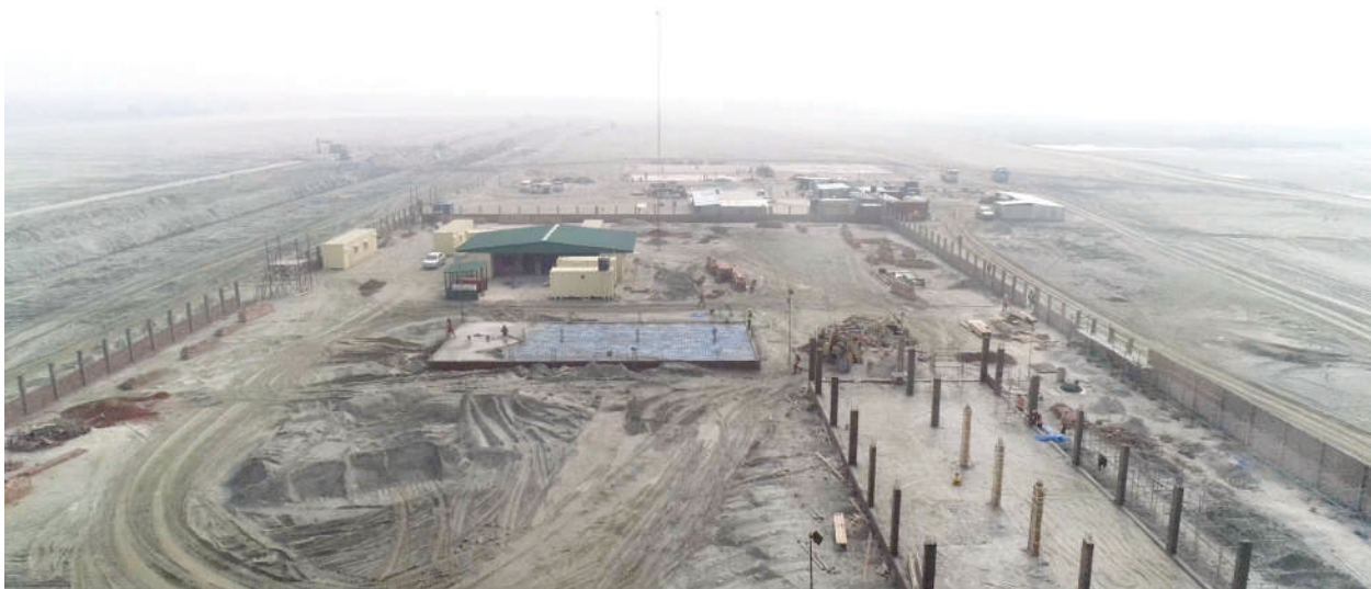
Aerial view of a construction of an Economic Zone. (Photo: Survey Team)
