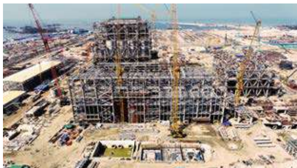
Project site under construction (Photo: JICA)
