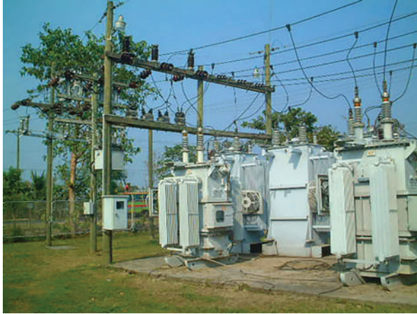
Rural Electrification Project (Photo: JICA)
