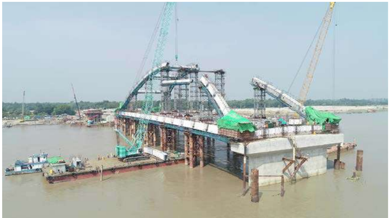
Kalna Bridge Under Construction (Photo: Tekken-AML-YBC JV)
