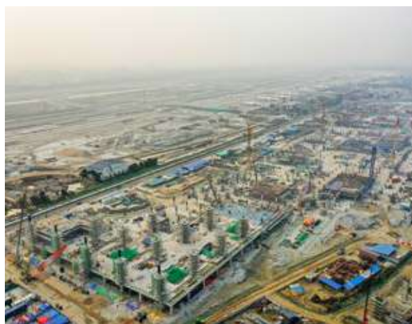
International Terminal 3 under construction (Photo: JICA)
