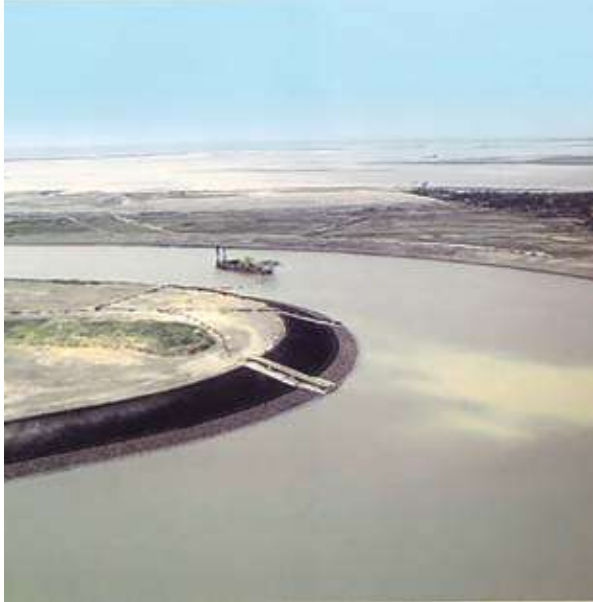
West Guide Bund (revetment embankment) of Jamuna Bridge (Photo: JICA)
