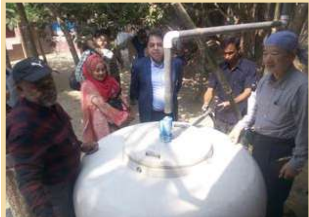
Installation of AMAMIZU (Photo: Institute for Sky Water Harvesting)
