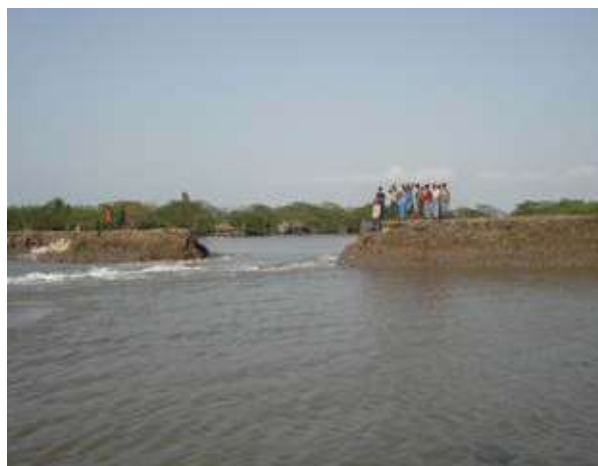
Embankment breached due to cyclone damage (Photo: JICA)
