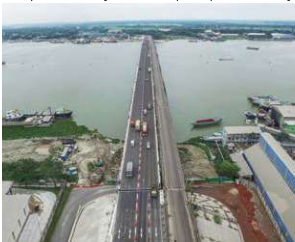
Meghna Bridge (Photo: JICA)
