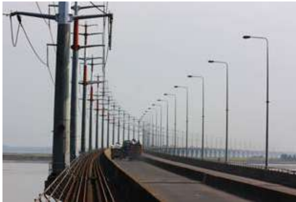
Jamuna Multipurpose Bridge. Around 11,000 vehicles cross the bridge every day. Trains, electricity, gas also go across the river on the bridge. (Photo: Masud Al Mamun)
