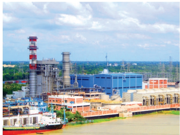
New Haripur Power Plant (Photo: JICA)
