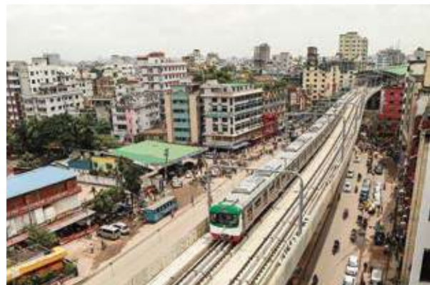
Test run status of MRT Line 6 (Photo: JICA)
