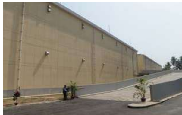
Ramp to access the second floor of the food storage (Photo: JICA)
