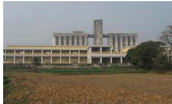
Panoramic view of the food warehouse constructed under the Food Reserve Capacity Enhancement Plan (2012). (Photo: JICA)
