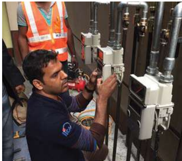
Installation scene of prepaid gas meter (Photo: ONODA.inc)
