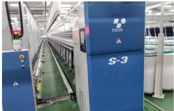
Spinning machinery installed by Energy Efficiency and Conservation Promotion Financing Project (Photo: JICA)
