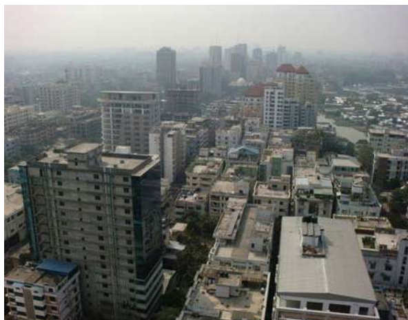
Dhaka City: Many buildings do not meet earthquake resistance standards. (Photo: JICA)
