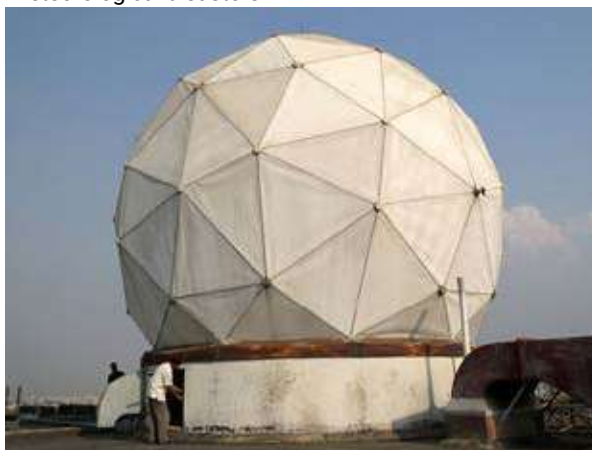
Dhaka meteorological radar station (Photo: JICA)
