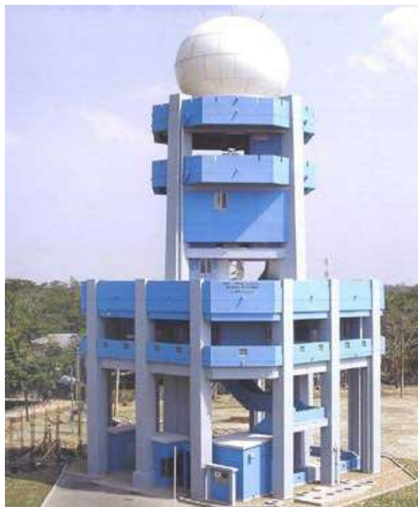
Khepupara weather radar (Photo: JICA)
