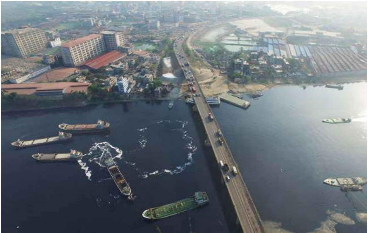
Meghna Bridge (Photo: OSJI Joint Venture)
