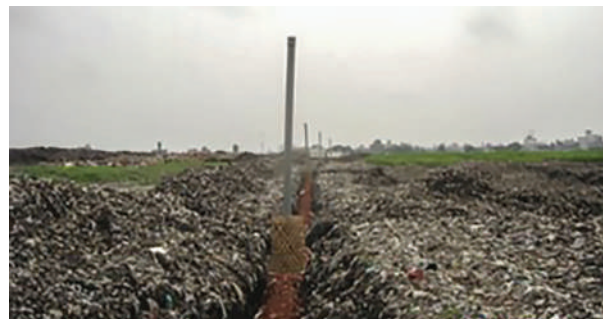
Current disposal site (landfill with gas treatment) (Photo: Yachiyo Engineering Co., Ltd.)
