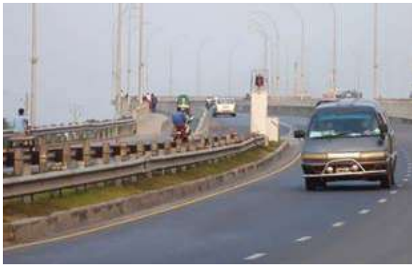
Rupsha Bridge (Photo: JICA)
