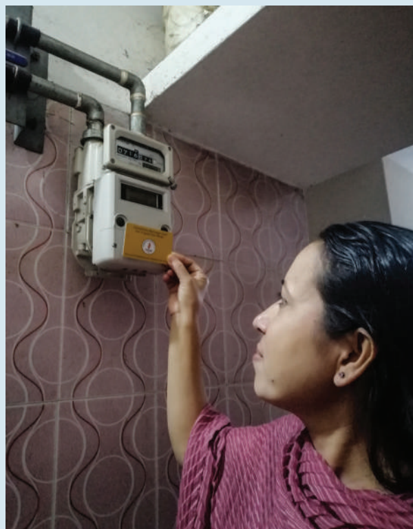
Prepaid gas meter introduced in Natural Gas Efficiency Project. Prepaid charge and download of consumed amount are done using IC cards. (Photo: JICA)
