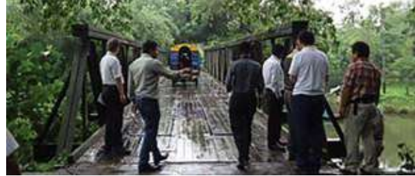
Bridge maintenance field survey (Photo: JICA)
