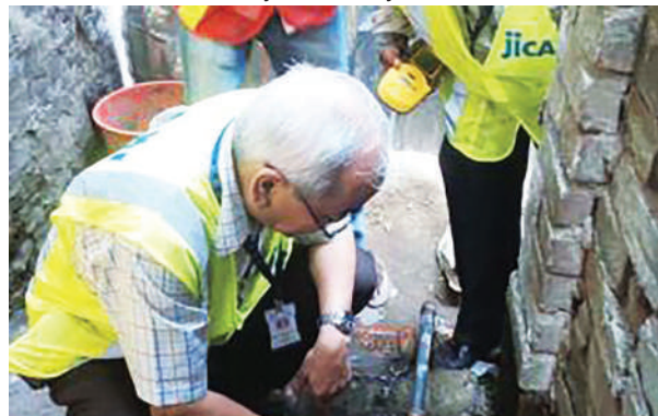
JICA expert checking water meter (Photo: JICA)
