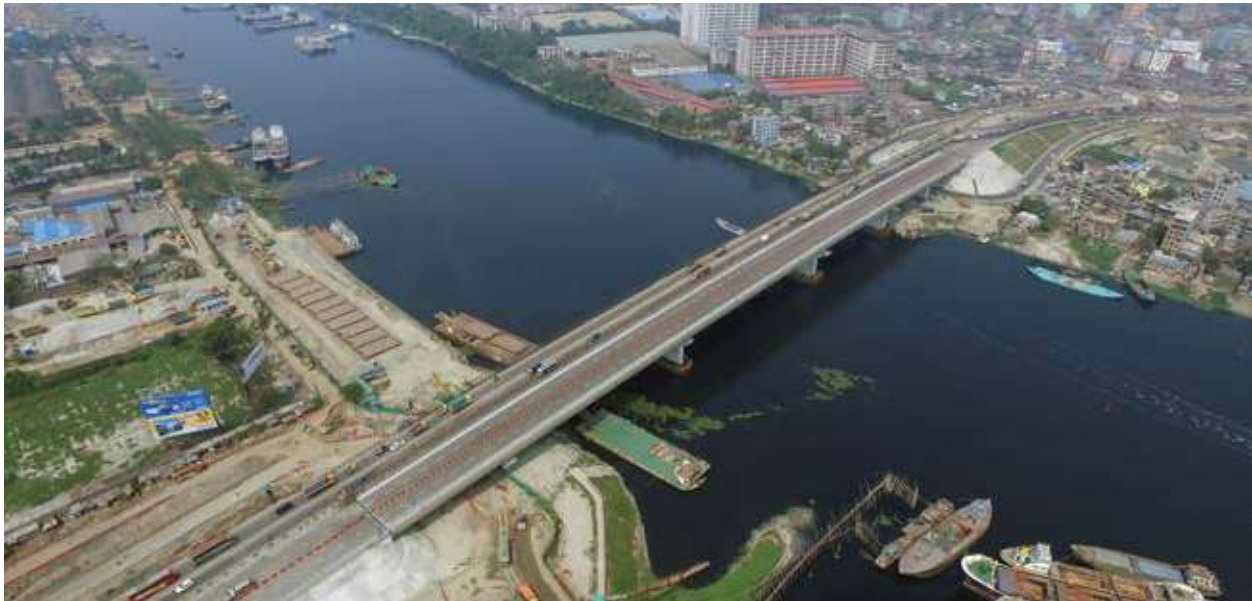
Kanchpur Bridge. (Photo: JICA)
