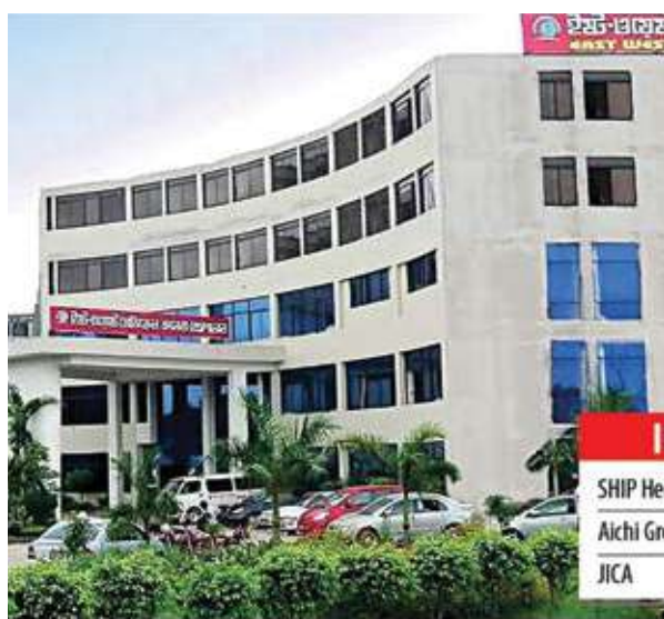
East West Medical College Hospital (Photo: JICA)
