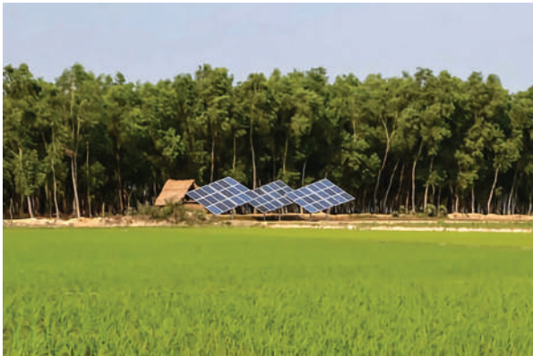
Renewable Energy Development Project is a two-step loan in which companies and general farmers use ODA loan funds through local financial institutions. This photo shows a solar power generation facility mainly used for irrigation pumps. (Photo: JICA)
