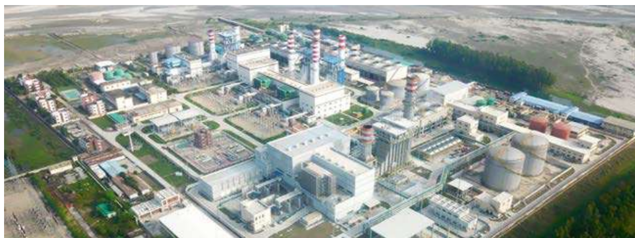
Sirajganj high-efficiency gas-fired power generation project (Photo: JICA)
