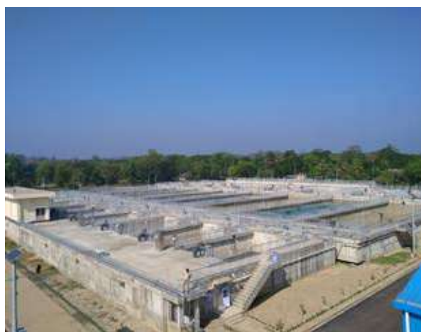
The Karnaphuli Water Treatment Plant under construction (Photo: JICA)
