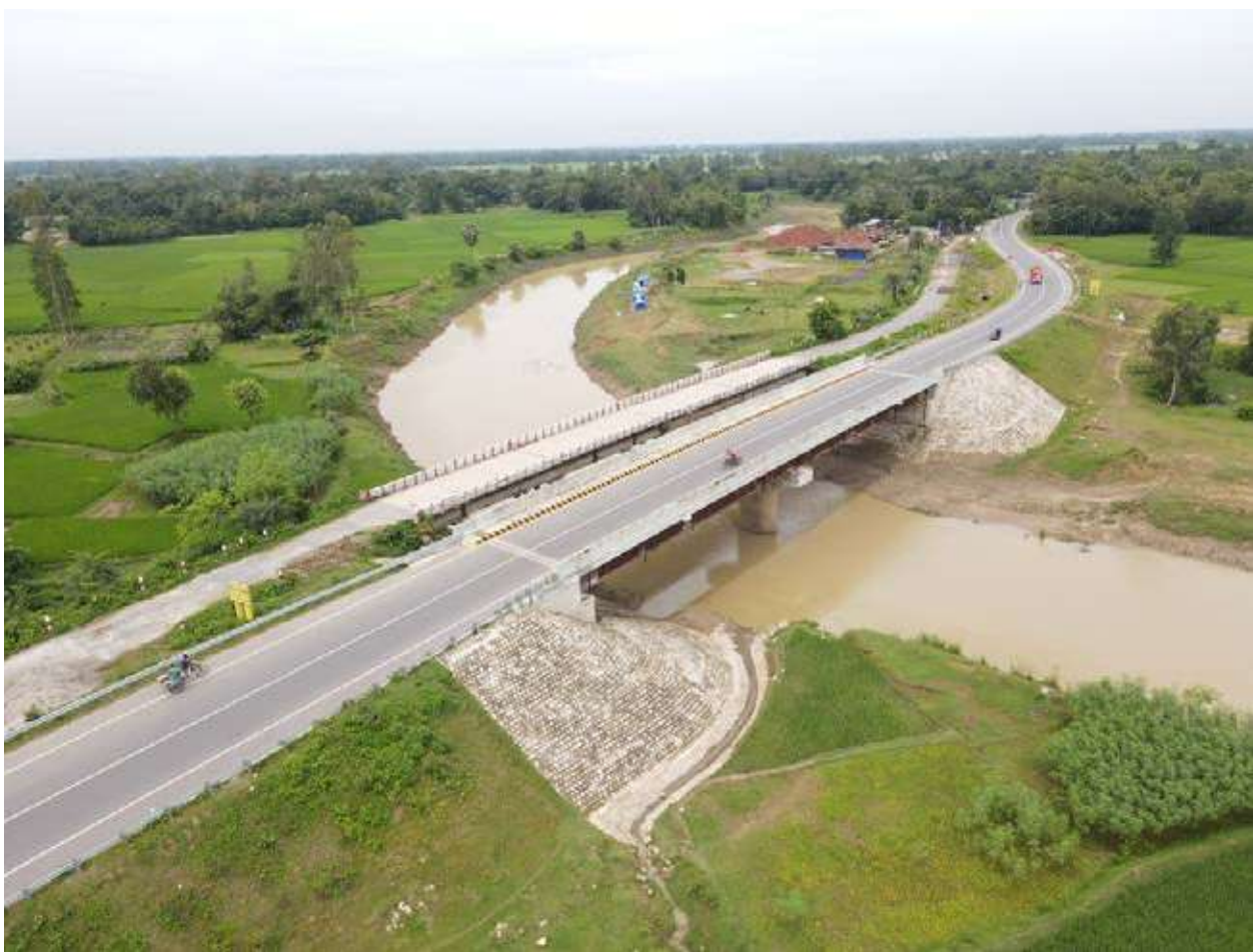
Bridges constructed in connection with connectivity enhancement (Photo: PW-02Contractor)
