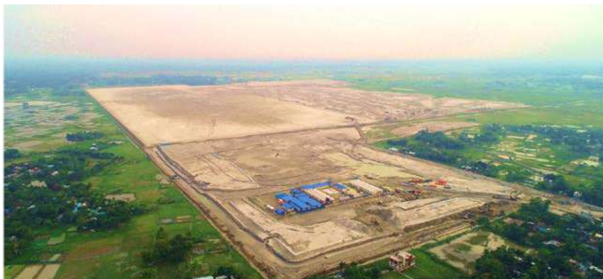
Project site under construction (Photo: JICA)
