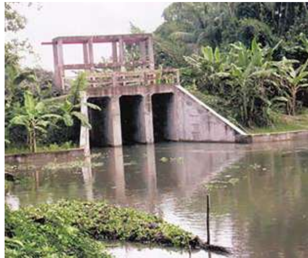
Sluice gate constructed by the Small Scale Water Resource Development Project (Photo: JICA)
