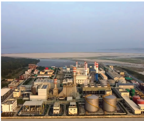
High-efficiency gas-fired power plant in Sirajganj (Photo: JICA)
