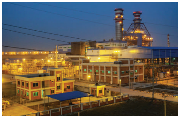
Bheramara Combined Cycle Power Plant. (Photo: JICA)
