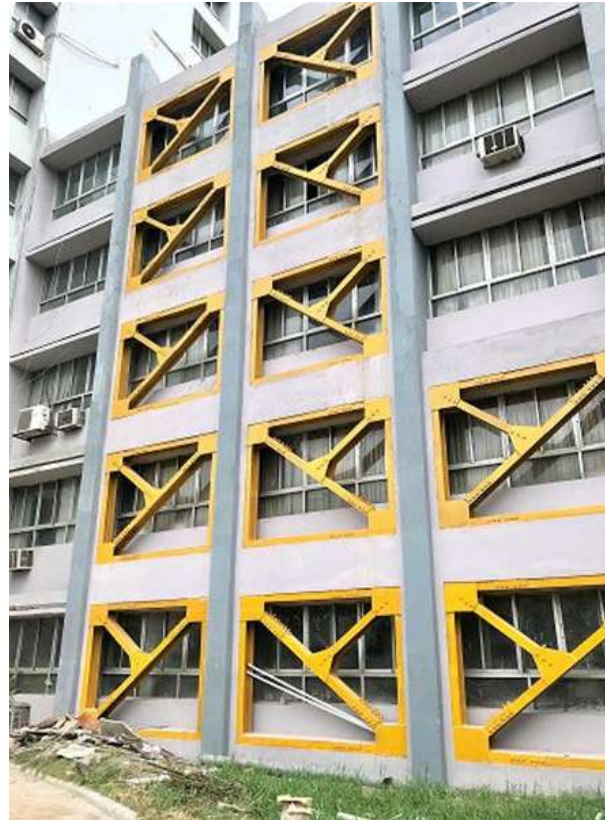
Building reinforced for earthquakes: Yellow steel bars are braces for anti-seismic reinforcement. (Photo: JICA)
