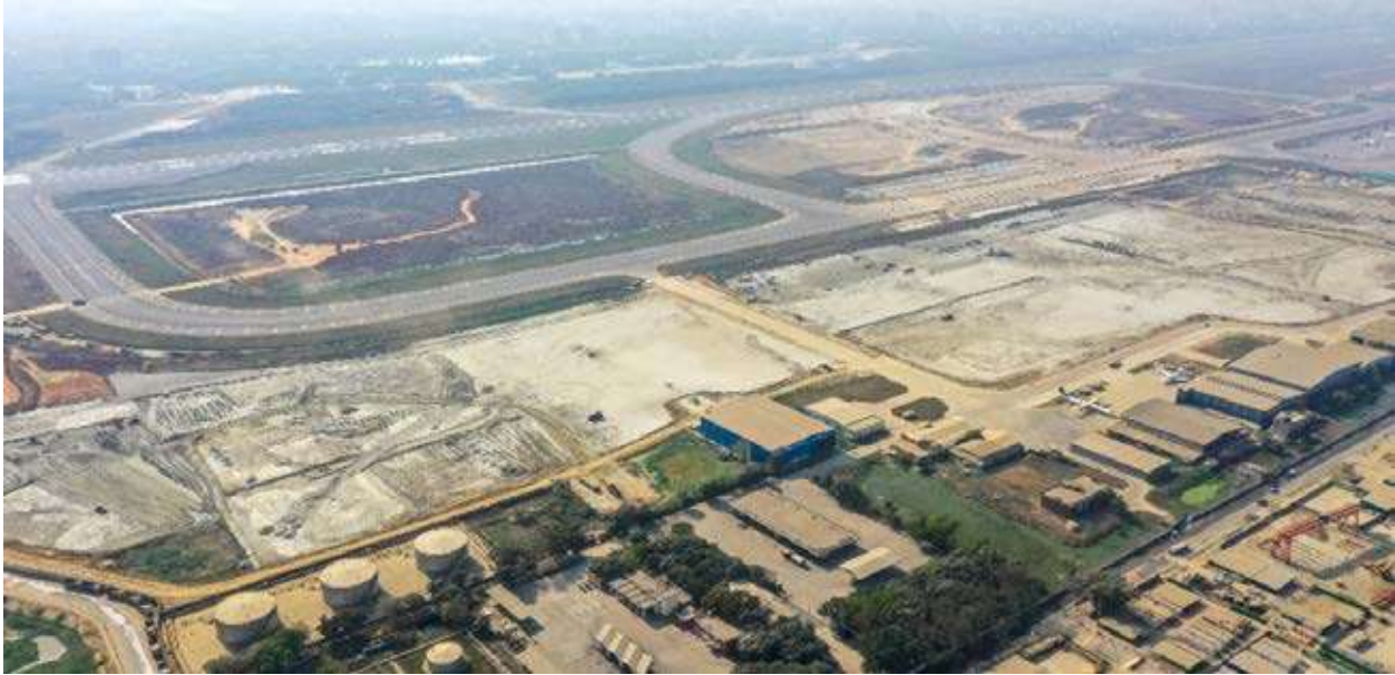
Dhaka Airport Terminal 3 construction site (Photo: JICA)
