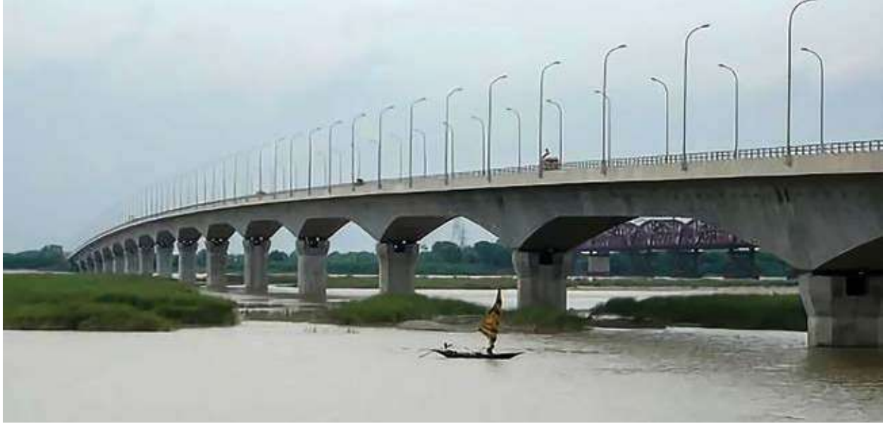
Pakshi Bridge (Photo: JICA)
