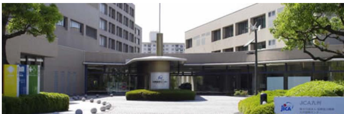
JICA Kyushu Main Entrance
