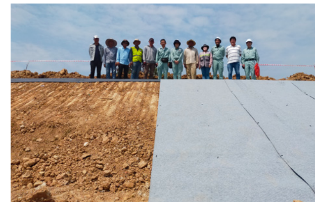
SDGs Business Validation Survey for Installation of Drainage Sheet to Prevent Rainfall-Induced Road Collapse in Cambodia implemented by Tanaka Co., Ltd
