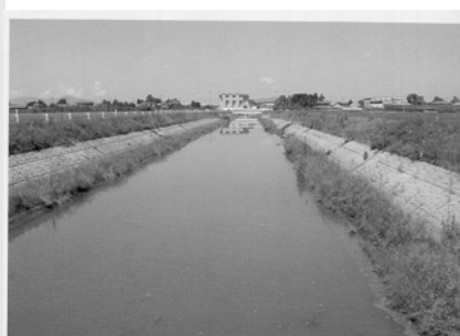
Main Drainage Channel
