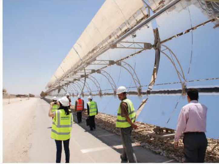
Kuraymat Integrated Solar Combined Cycle Power Plant ] Project (completed in 2011)
