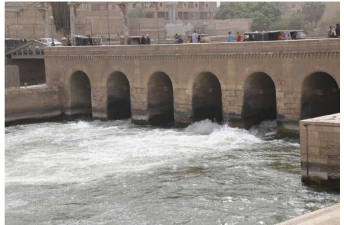
Water flow from Existing Regulator
