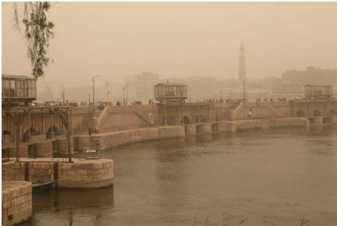
Existing Dirout Group of Regulators
