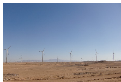
Zafarana Wind Power Plant
