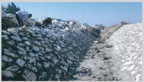
Joint Repair work in Damietta
