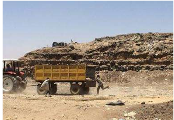
Waste Management: Promoting improvement of final disposal sites to realize a Clean City (Sudan)
