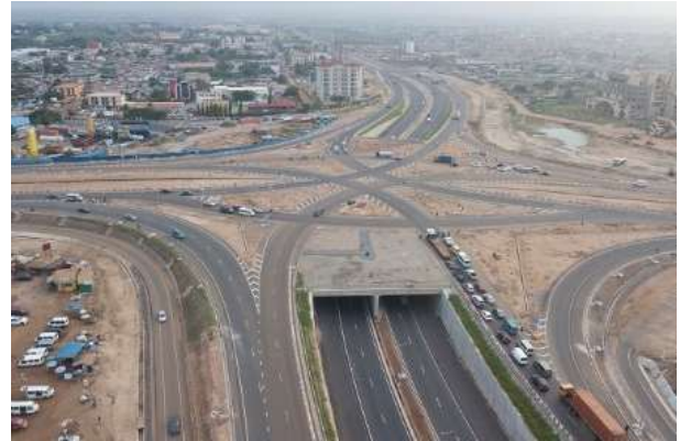
The Tema Motorway Interchange, with the largest underpass in Ghana. Constructed under the "Project for Improvement of Ghanaian International Corridors"
