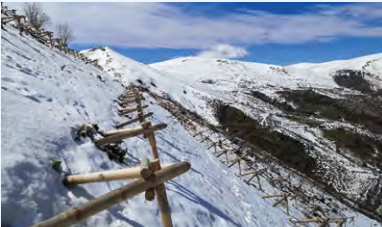
Wooden frames installed and trees planted to prevent avalanches, one of the main natural disasters in Kosovo.
