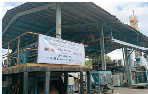
Kluang Pilot Plant, which produces biomass pellets
