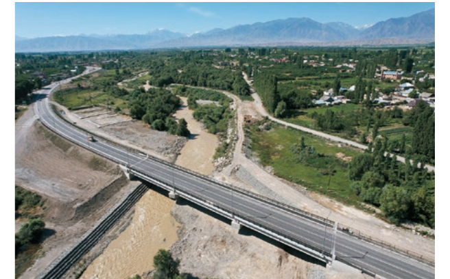
The rebuilt Urmalar River Bridge (Sakura Bridge)
