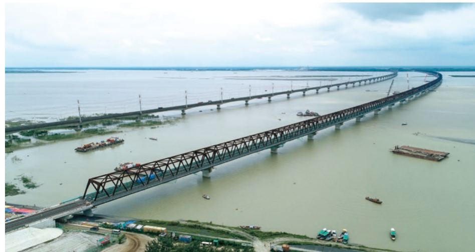
Jamuna Railway Bridge, the longest in Bangladesh, commenced operation in March 2025 [Photo: OTJ Joint Venture (Obayashi Corporation, Toa Corporation & JFE Engineering)]
