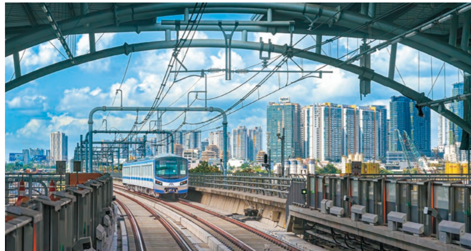
Ho Chi Minh City Urban Metro Line No.1 commenced operation, including the first underground section in Vietnam
