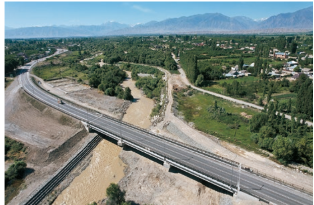
The rebuilt Urmamal River Bridge (Sakura Bridge)
