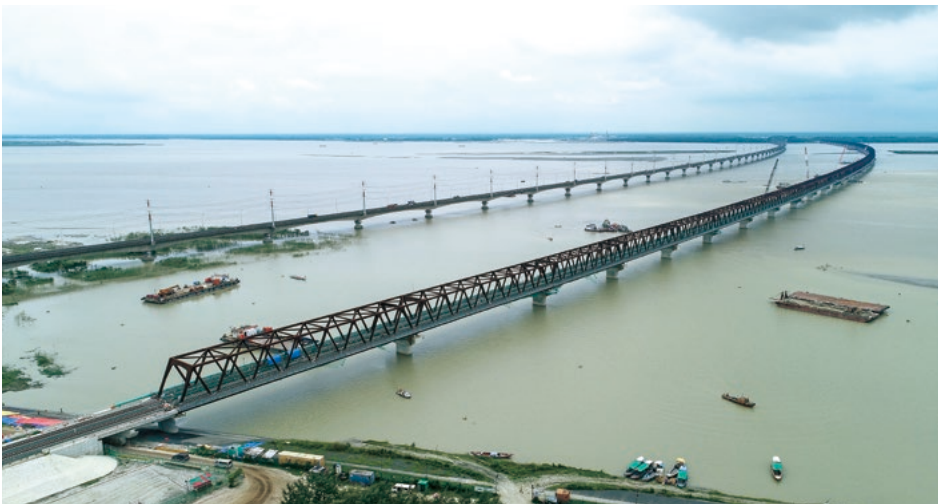
Jamuna Railway Bridge, the longest in Bangladesh, commenced operation in March 2025 [Photo: OTJ Joint Venture (Obayashi Corporation, Toa Corporation & JFE Engineering)]
