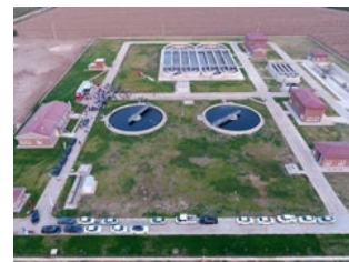
Sewage System (image by JICA)
