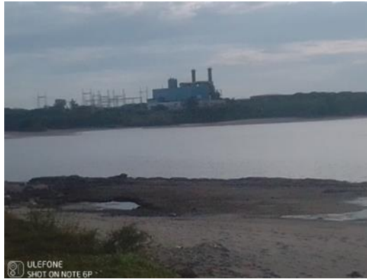
Figure 16-1 Thermal power plant (GEOSA)
