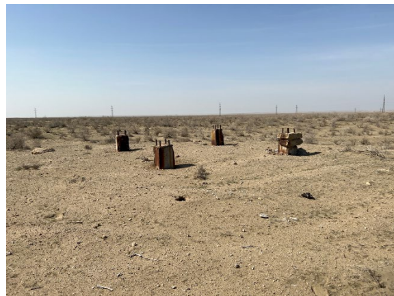
Figure 6: Remains of the OHTL foundations on the Project site
