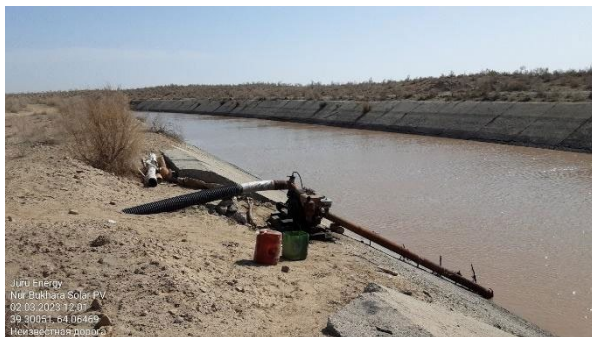
Figure 38: Photo of pump
