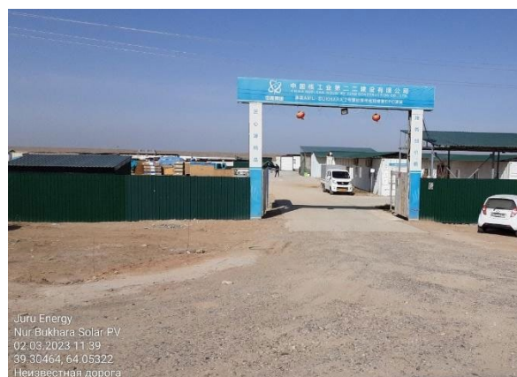
Figure 49: Workers' temporary camp
