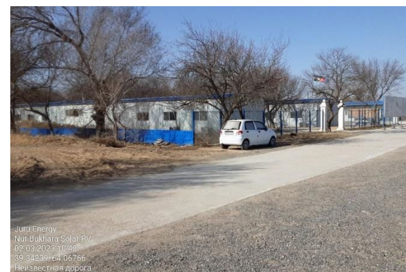
Figure 47: Workers temporary camp
