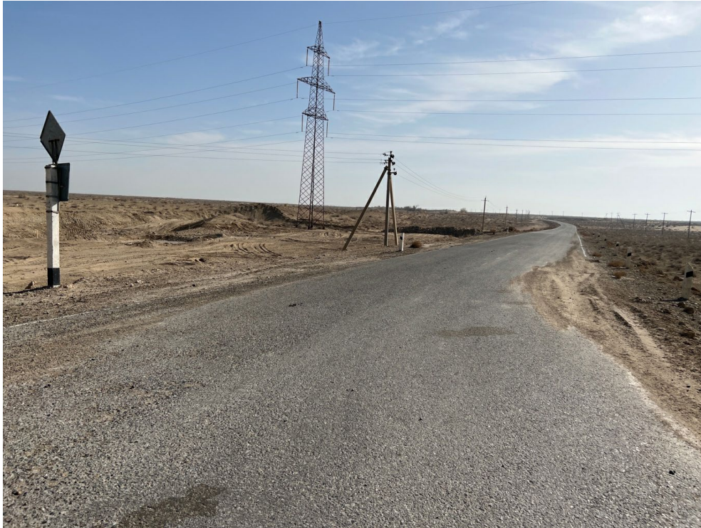
Figure 21: Existing R78 (photo)
