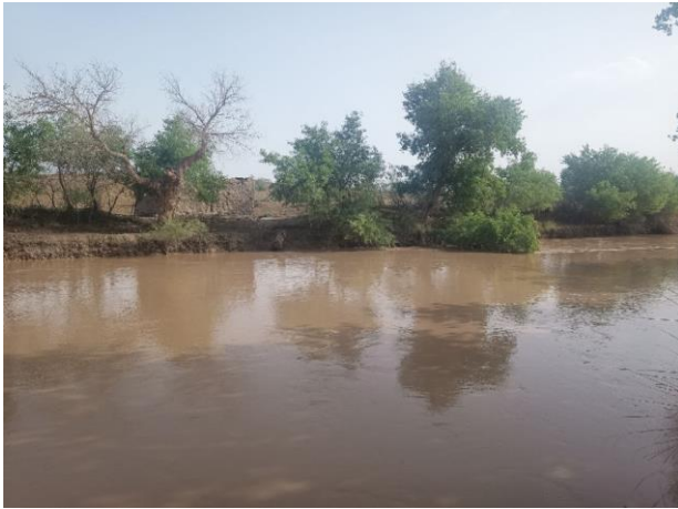
Figure 2: ABIS canal with open water, trees and shrubs
