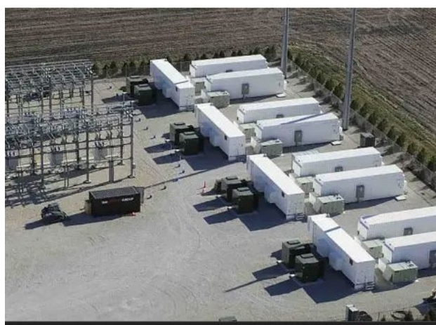
Figure 9: Typical container BESS (external) 1 :
