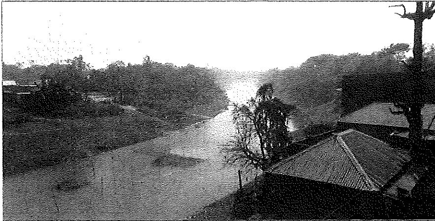
Figure 11: Bridge No. 23 over River Boral (view from Downstream) showing Stable Bank
