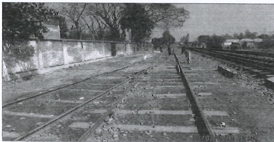
Figure 7: Fertiliser Godown and Boundary Wall
